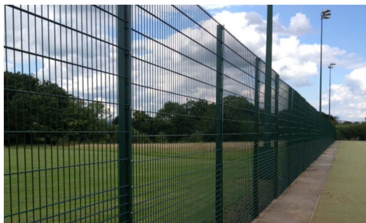
Example weld mesh fencing
